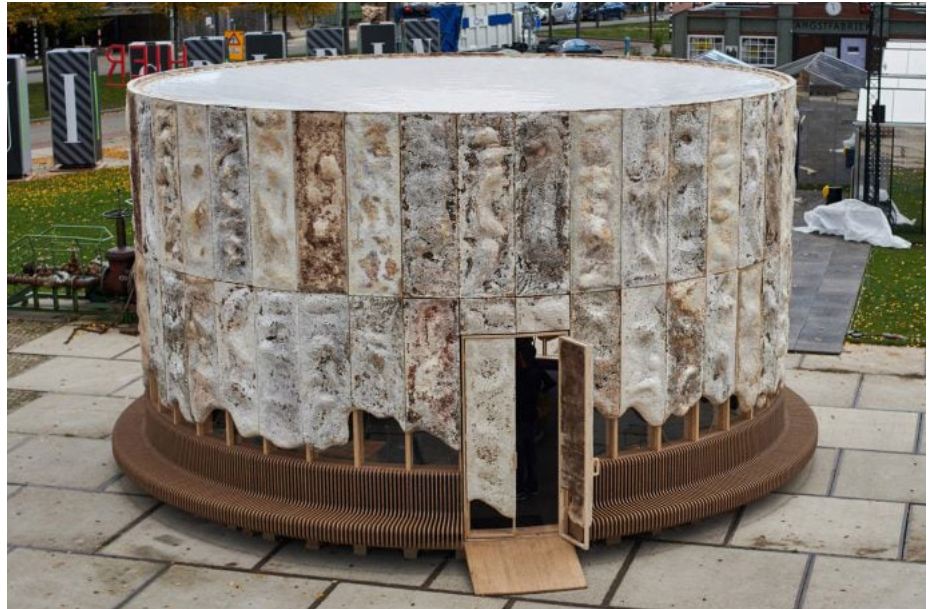
Mushrooming: The Growing Pavilion, a building made from mycelium, cleans the air as it grows.
